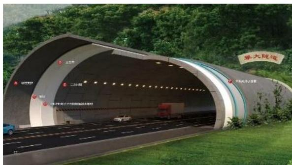
waterproof construction. Oriental Yuhong's HDPE polymer self-adhesive waterproof membrane effectively solves the project's waterproofing challenges with its excellent properties such as pre-paving anti-seepage, flameless construction, lightweight, and easy installation, contributing to the high-quality construction of the project.
